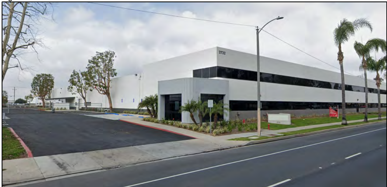
Figure 31: 2700-2722 South Fairview Street – Street View
